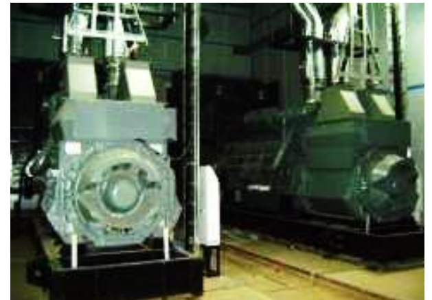
● DG (placed in the basement)
